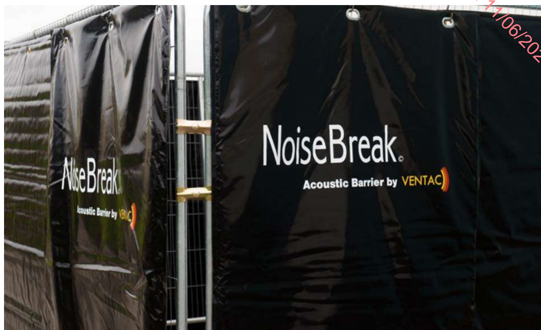
Figure 12--: Temporary Construction Noise Barrier © Ventac
